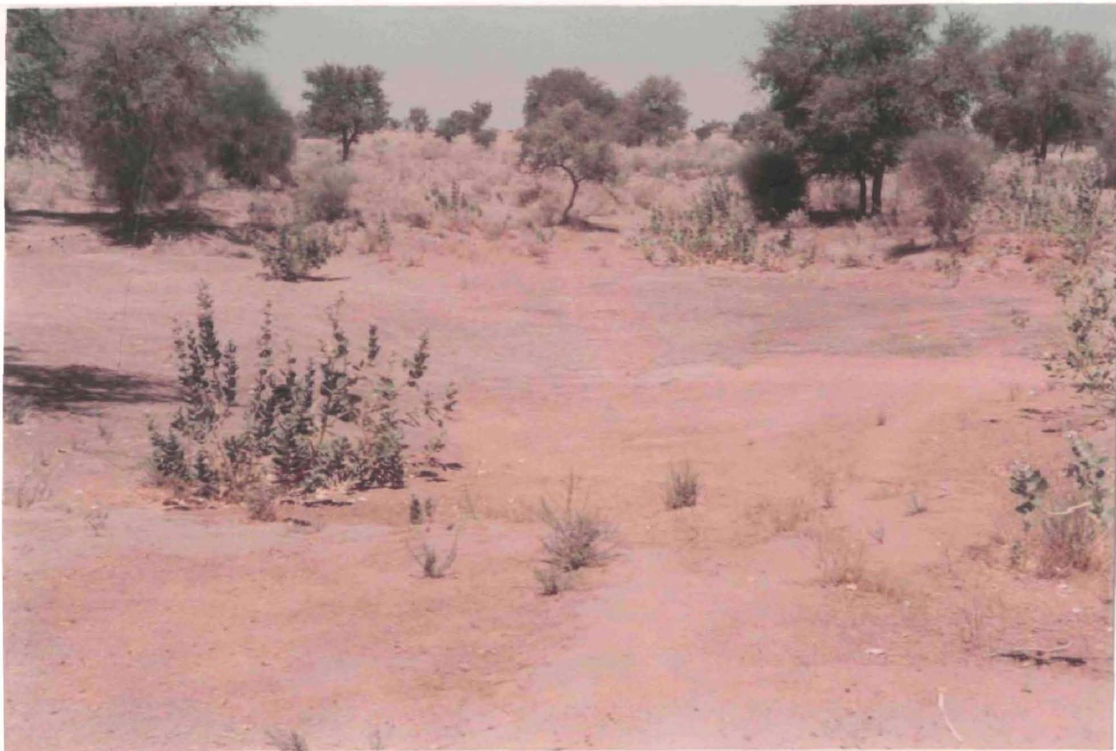
Plate 5. Silting of the nadi resulted in the reduction of its water storage capacity
